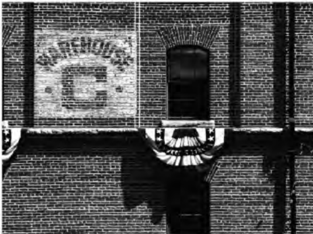
WAREHOUSE C, ORIOLE PARK AT CAMDEN YARDS
